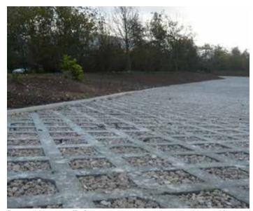
Permeable paving (Reference: www.externalworksindex.co.uk).
