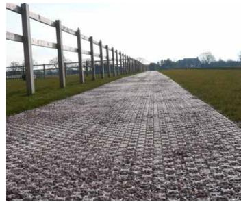
Permeable paving using gravel paver material (Reference: www. terram.com).
