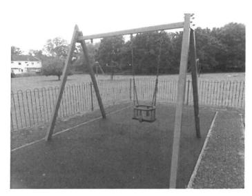
One swing seat has been removed some time ago. The frame is too worn and cannot be repaired for swing to be replaced.
