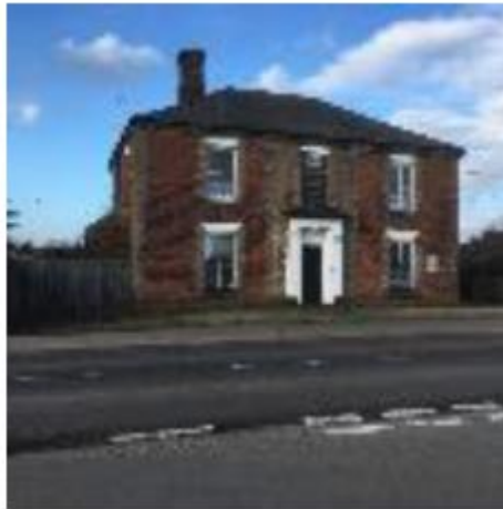
Former Railway Hotel
