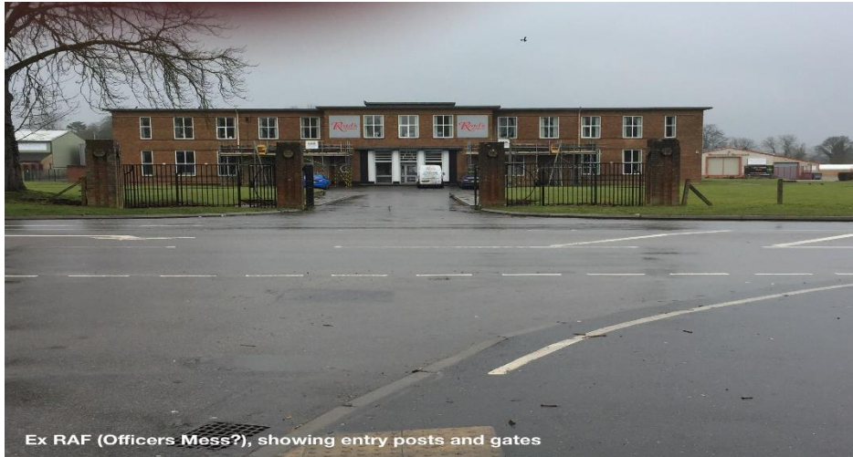
Entrance to site and Ventura House
