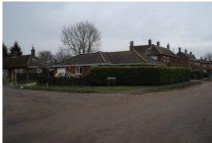
New Build on West Road
