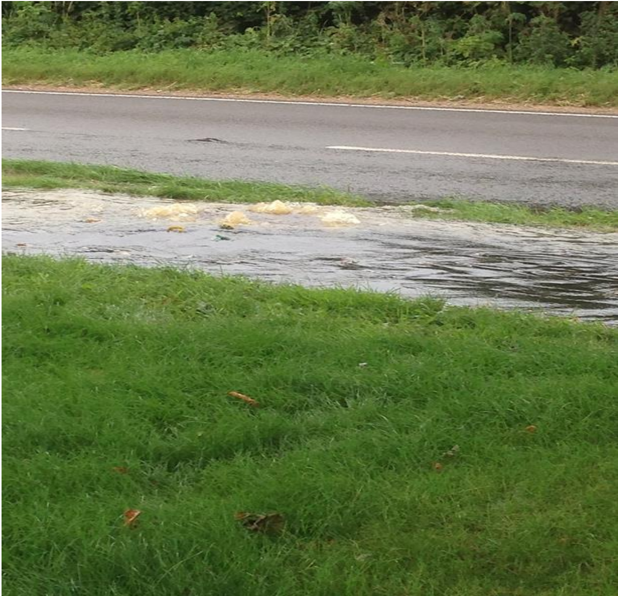
Foul sewer on Thetford Road surcharging
