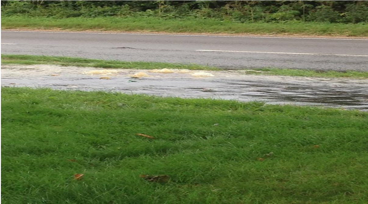
Foul sewer surcharging on Thetford Road
