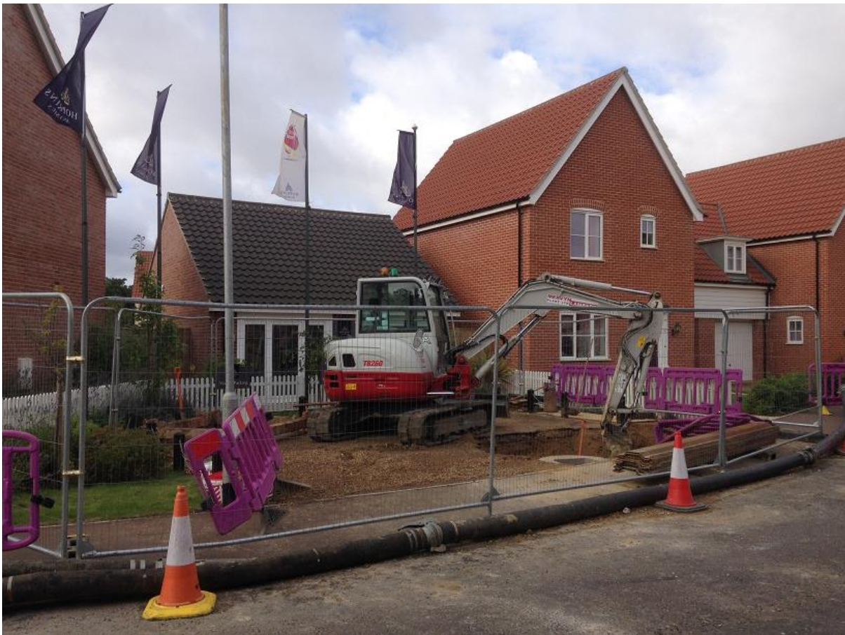
Anglian Water over pumping past the collapsed drain
